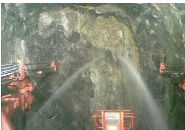
**Fig 4** Water ingress along sub-horizontal joints
